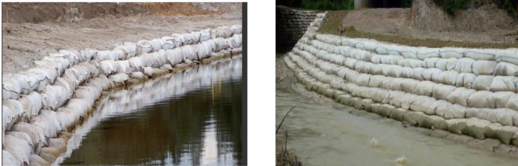
Figure 11: Pictures of some projects implemented with geotextile bags reinforcing the tendencies of the channels
