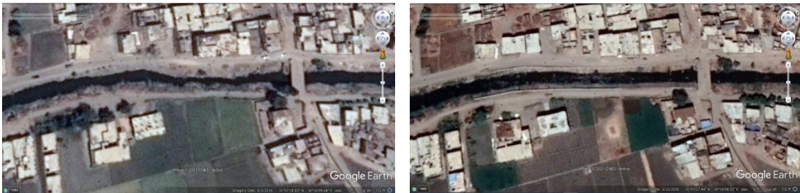
Figure 25: Izbet Al-Tawala sector, before & after protection works from google earth
