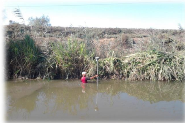
Figure 4 : Surveying works of Abu Hummus Drainage sectors
