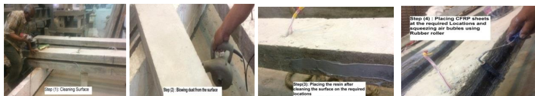
Fig. 5: Steps of strengthening technique
