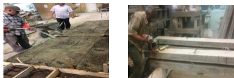
Fig.4: Mechanical compaction and surface preparation
