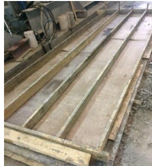
Fig. 2: Wooden formwork
