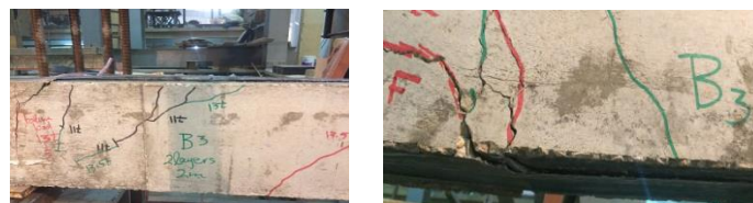
Fig. 9g: the mode of failure for Specimen B3
