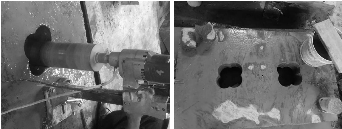
Fig. 1: construction of the openings using drilling core machine.
