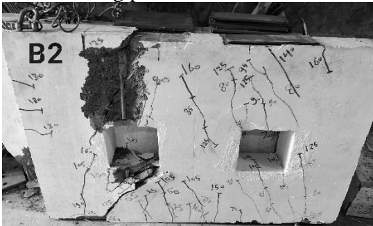
a- Cracking patterns of B2 after failure
