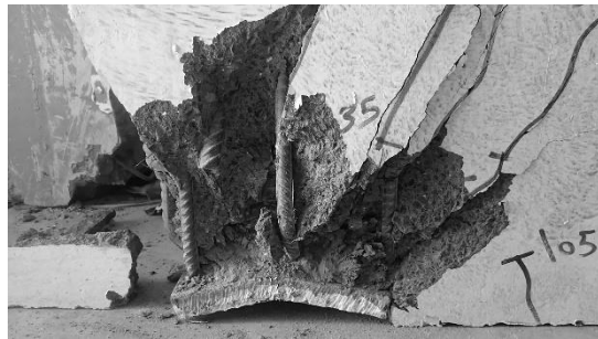
b- Bearing failure of B1
