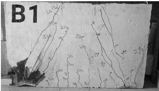
a- Cracking patterns of B1 after failure
