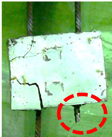
(a) Rupture of reinforcing steel bars of for S-P-05d.
