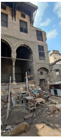
(a) General view of the structure.
